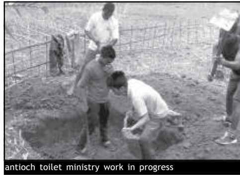
antioch toilet ministry work in progress
